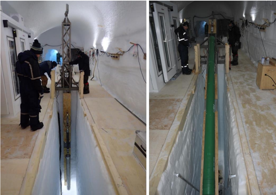
The final reaming and casing installation was conducted using the deep winch and tower apparatus, May, 2017.
