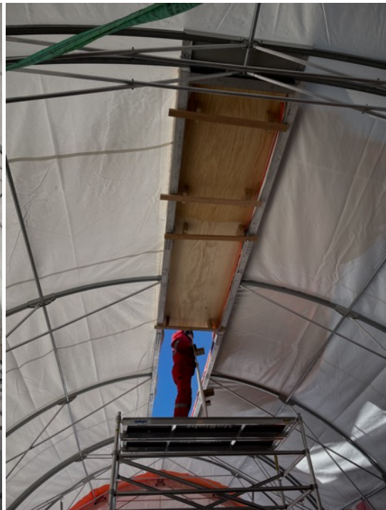
The scaffold is needed for closing the roof of the drilling tent. Photos by B. Seth
