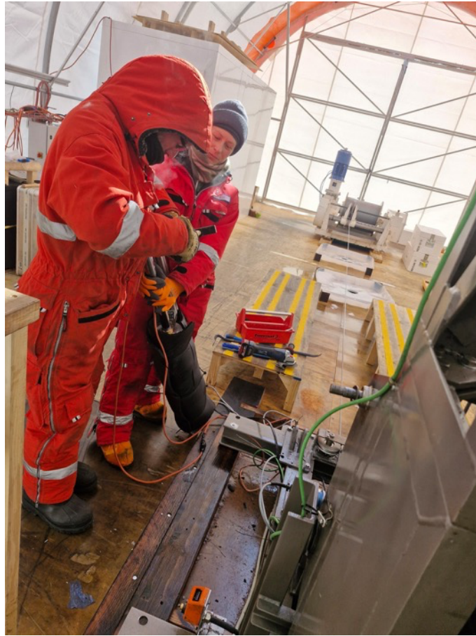
Repairing one of the tower actuators. Photo by H. Traeger
