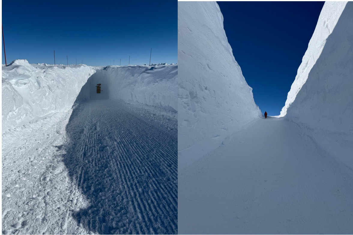
The storage cave near Concordia Station. Behind the small door on the left is the entrance to a snow cave, approximately 40 meters long, where the Beyond EPICA samples are stored for the future. On the right is the view from the bottom of the ramp. Photo by C. Barbante.
