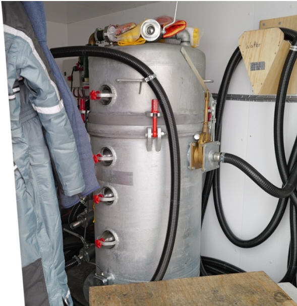
The chips melting system, referred as "the pig". Credit: F. Wilhelms ©PNRA/IPEV
