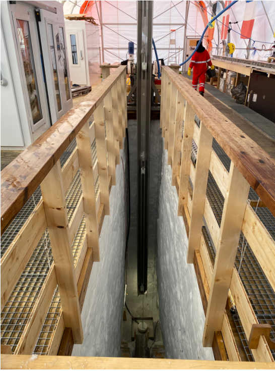
Figure 1: The impressive tilting trench: photo: O. Alemany
