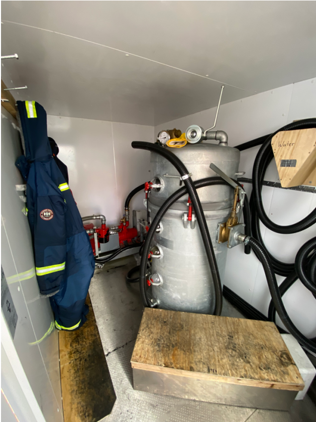
Figure 1: The "pig" where we are separating drilling fluid from water : photo: O. Alemany
