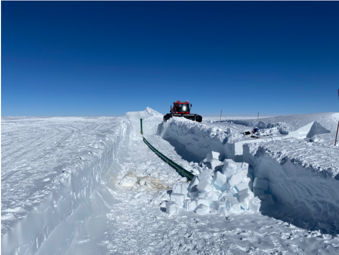
Figure 2: Finishing the ventilation to cool the science trench: photo O. Alemany
