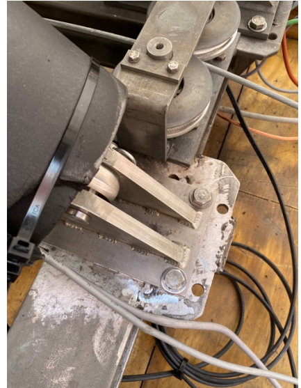
Figure 2: the repaired weldment on the mast frame
