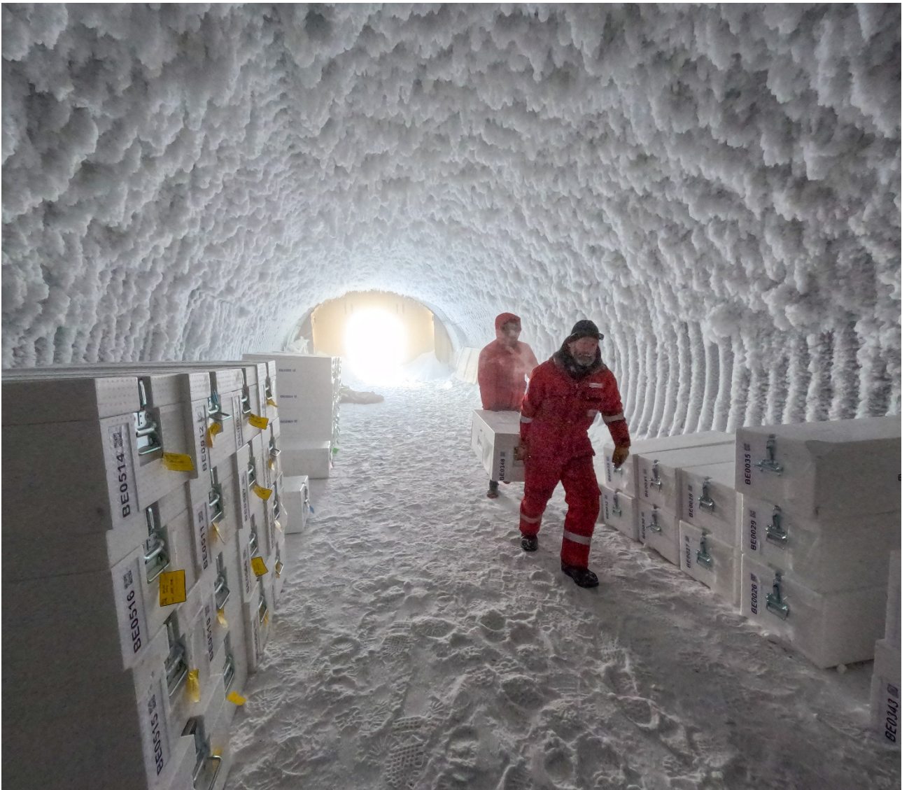
Markus and Lemmie carry an ice core box from BELDC into the Tubosider storage cave at Concordia Station. The tunnel is about 10m under the surface, and maintains a year-round temperature of around -50°C. The boxes on the right are ready for processing, while those on the left have been worked on sit on the left ready for shipping to Europe. (Photo: Mulvaney, GoPro Hero11, 3mm, 1/160, f2.5, ISO1000)
