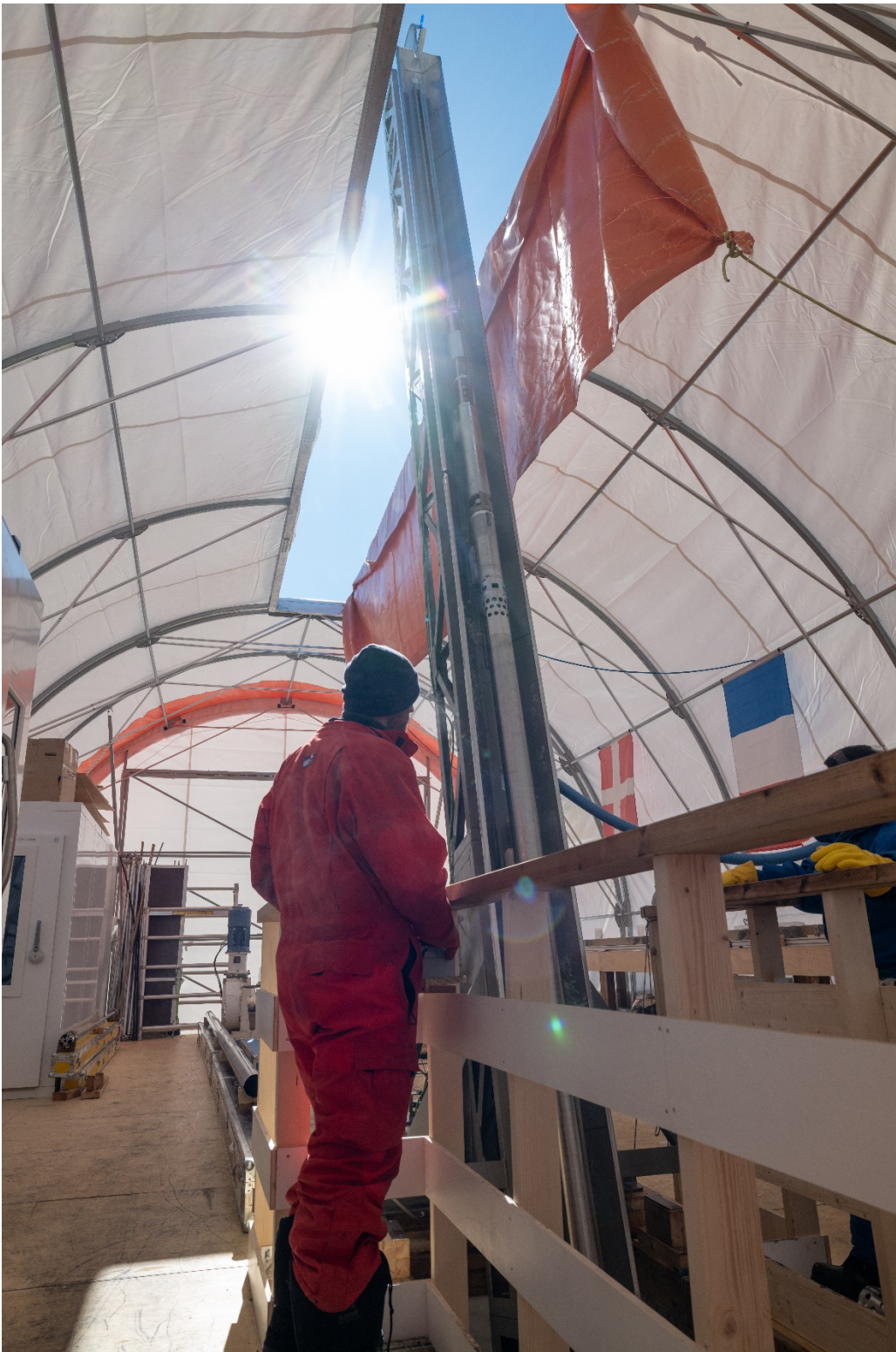
Martin raises the mast and drill from the horizontal to the vertical, in the midday sun, ready to send the drill down the borehole. (Photo: Mulvaney, Leica SL2, 24mm, 1/800, f8, ISO400)
