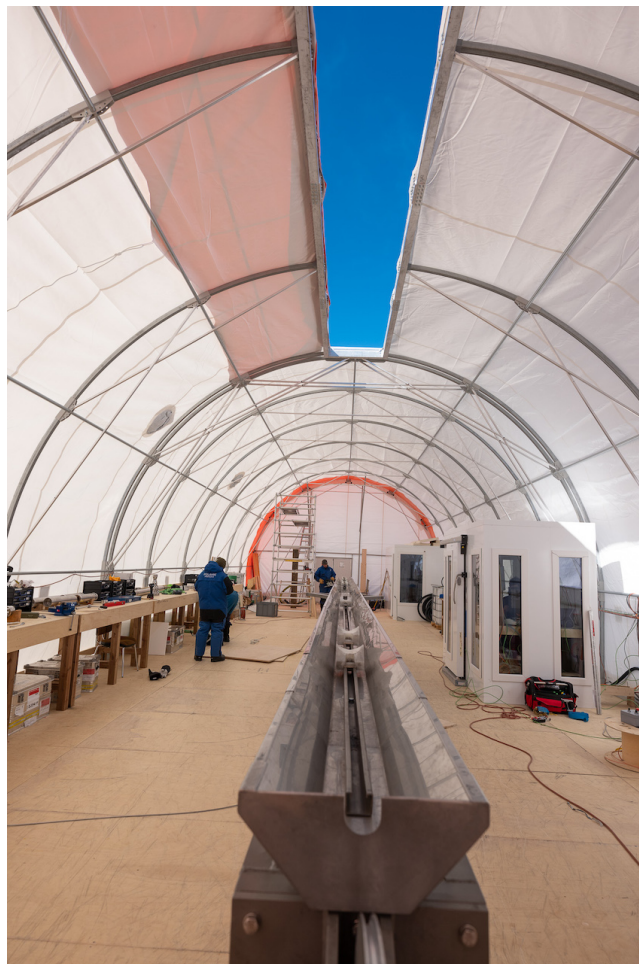
View along the drill tower through the BEOIC drill tent with the open roof, the driller's cabin and the fluid recycling cabin along the right side of the tent. Photo: T. Stocker (Leica SL2-S, 20 mm, f 5.6, 1/800 s, ISO-400).
