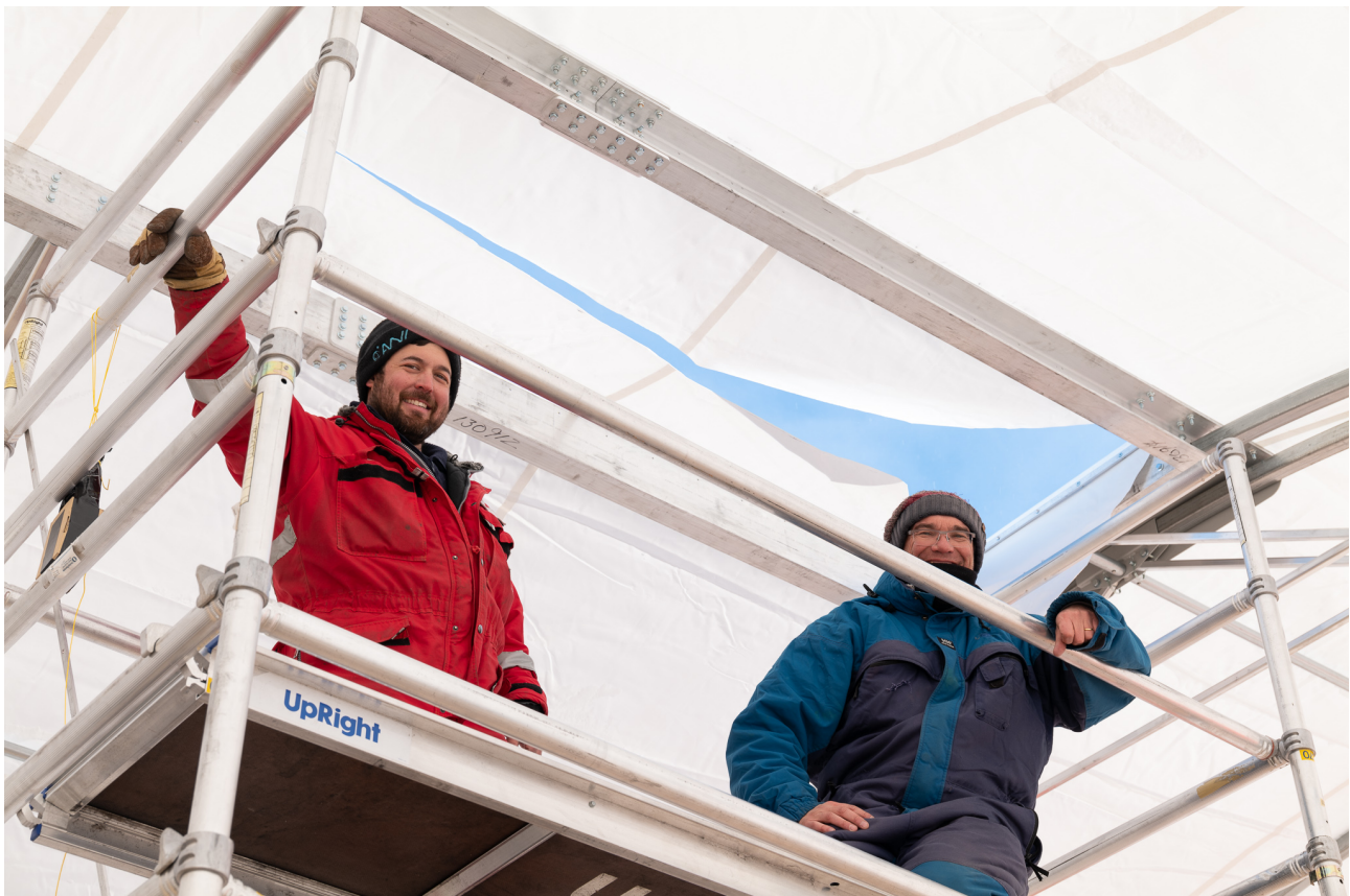
Matthias and Olivier on the scaffolding cutting through the tent canvas.
