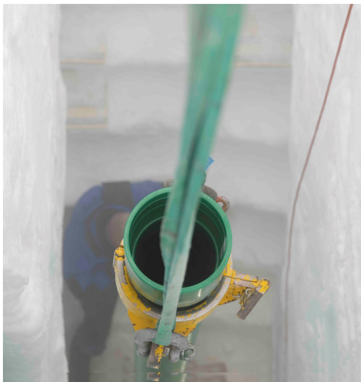
December 23, 2021: Setting the last BEOIC casing tube. Photo: T. Stocker (Leica SL2, 90 mm, f4, 1/200, ISO 100)
