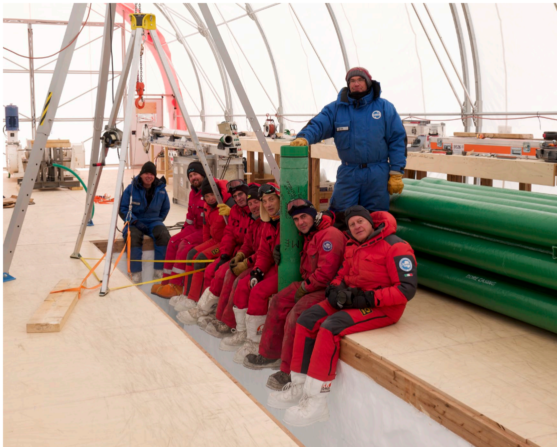
In the preparation of the casing operation at the BEOIC drilling trench.
