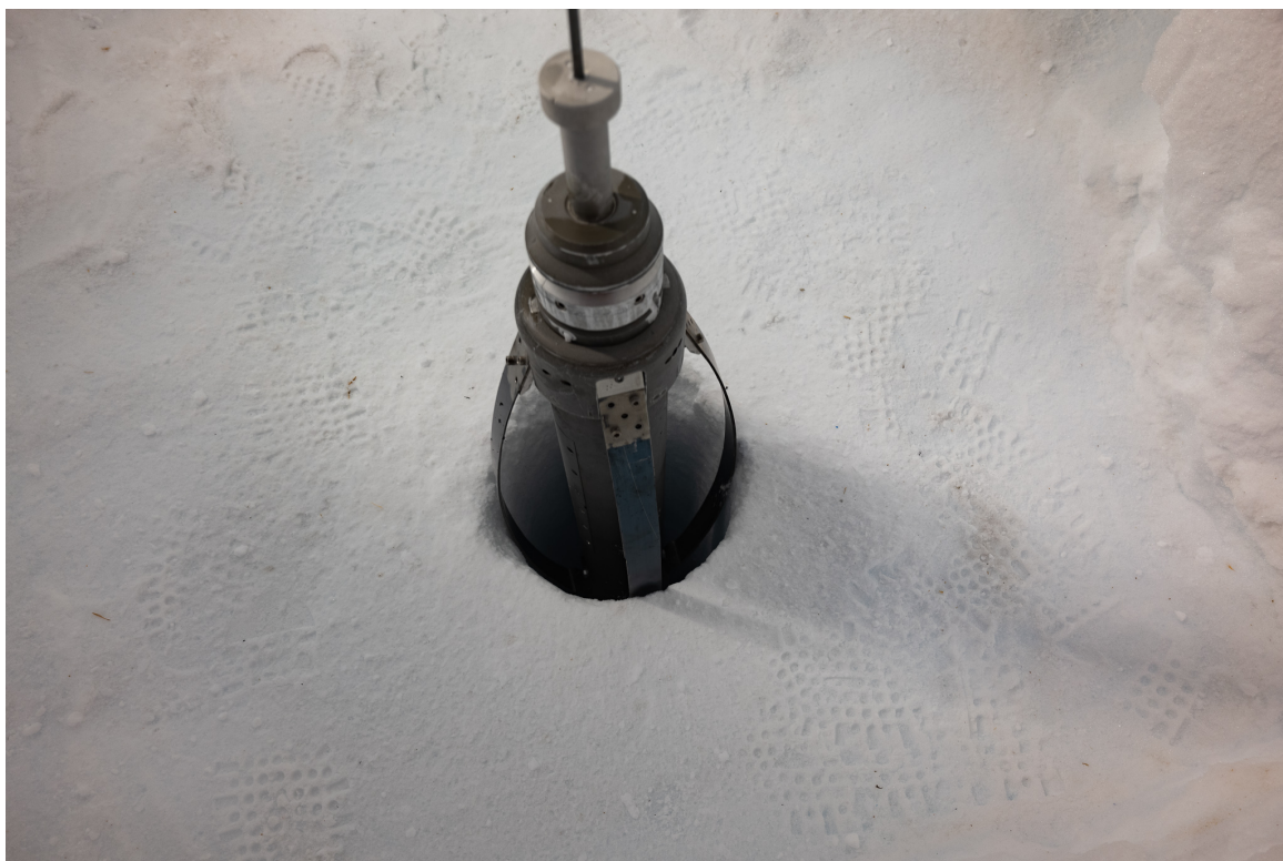
The IGE reamer entering the BEOIC hole at the drilling trench floor at about 8 m depth.
