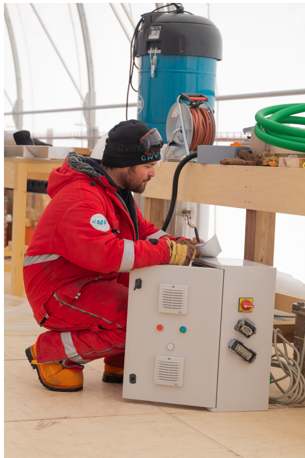
Matthias working on the electrical installation in the drilling tent.
