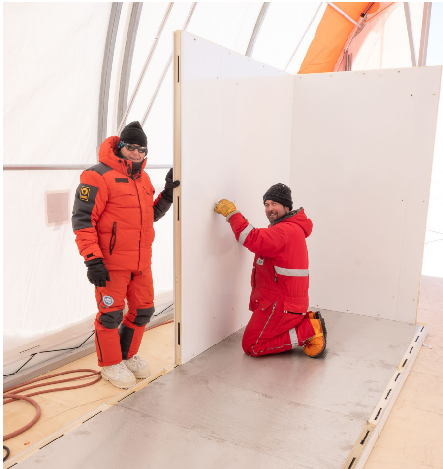
Carlo and Mathias assembling the Vissmann elements. Photo: T. Stocker
