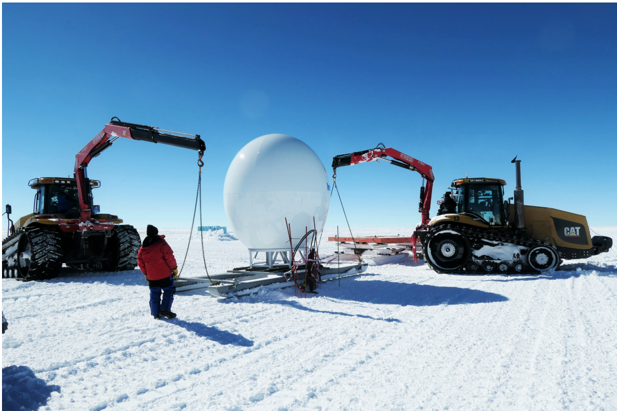
Placement of the antenna for broadband communication. Photo: T. Stocker
